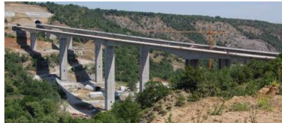
Fig 1: View of the viaduct
